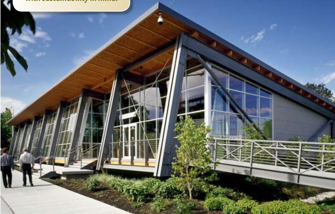
*The Discovery Center features bioswales and a permeable paver parking lot to protect Lake Union water quality.*
